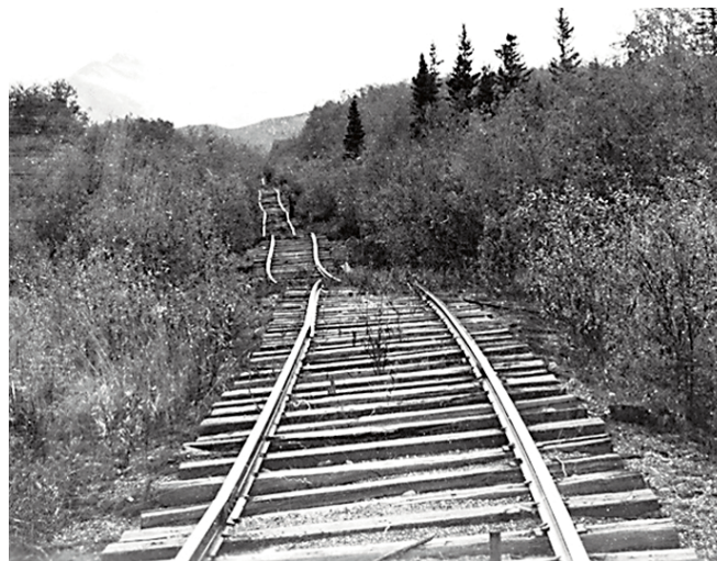
Figure 2.2 Damage caused by permafrost subsidence (USGS, 2002)
